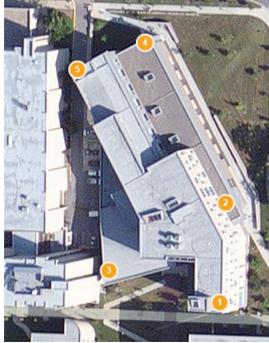
Figure 8. Indoor Testing Area [17].
